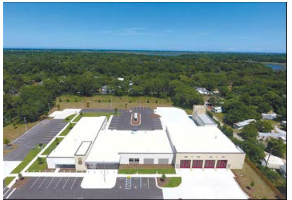
Current Station 5, which the new Station 22 in Silverleaf will be modeled after.
