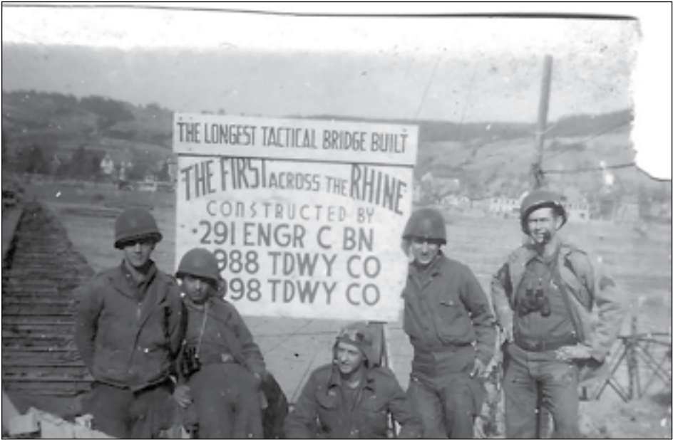
Allied soldiers rapidly construct a pontoon bridge across a European river. Spates's 291st Engineers, Company C, performed this critical, high-pressure work at locations like Remagen to keep troops moving forward.
